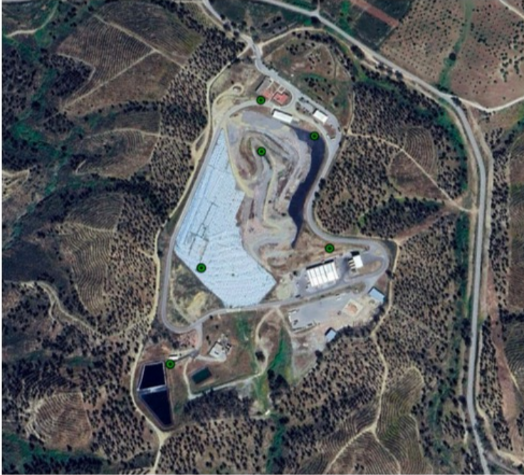
(a) Legal landfill site.
